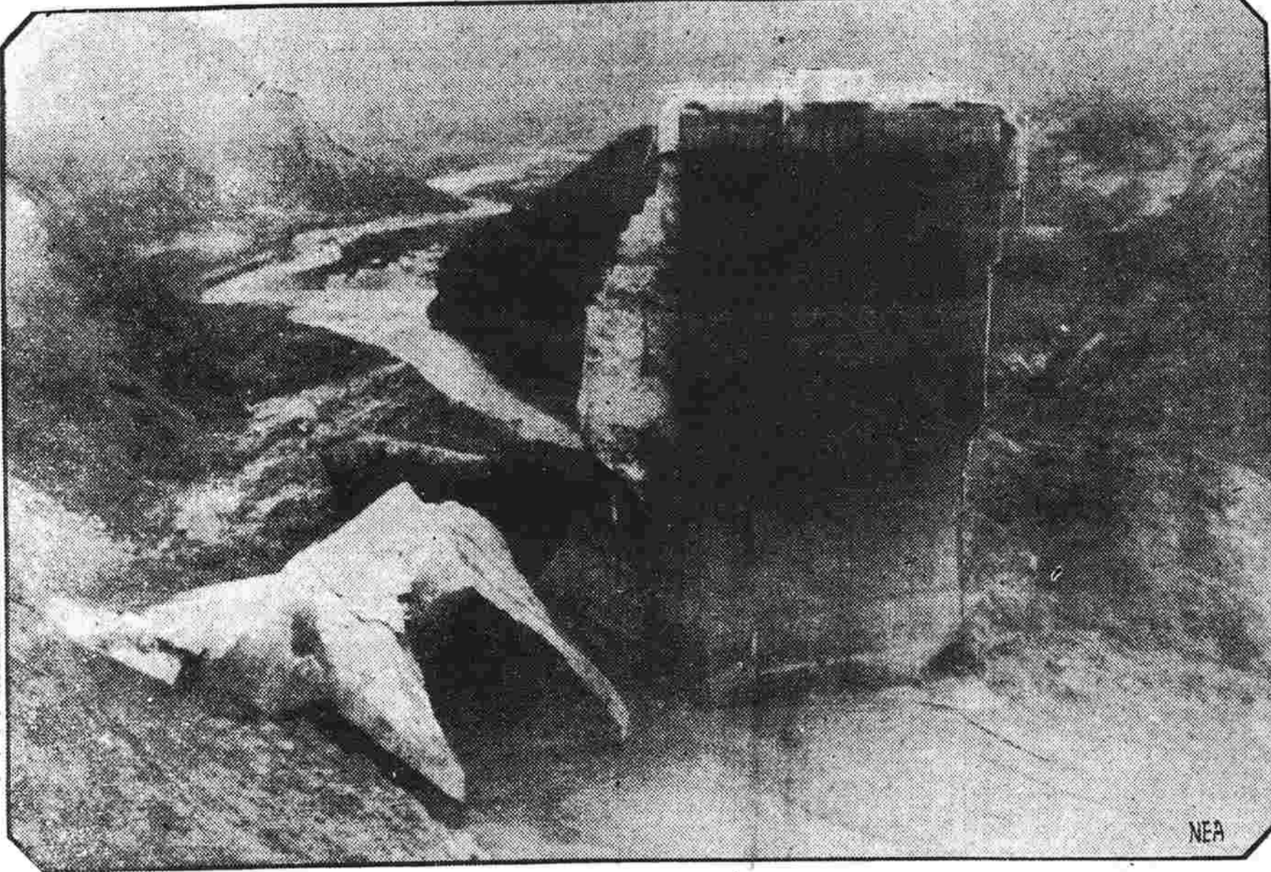
Here is an air picture of the ruins of the great St. Francis Dam near Newhall, California, after it burst and sent a torrent down the tranquil Santa Clara River Valley. Breaking of the dam, caused by a cloudburst, released 38,000 acres of impounded water. Death and destruction rode the crest of the flood. Of the dam, only the concrete monolith shown in the center of the photo was left. The picture was taken by an NEA Service photographer from an airplane and telephotated to New York from Los Angeles.
